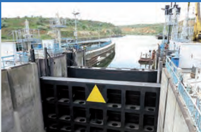
Hubtor - Vertical Lift Gate
