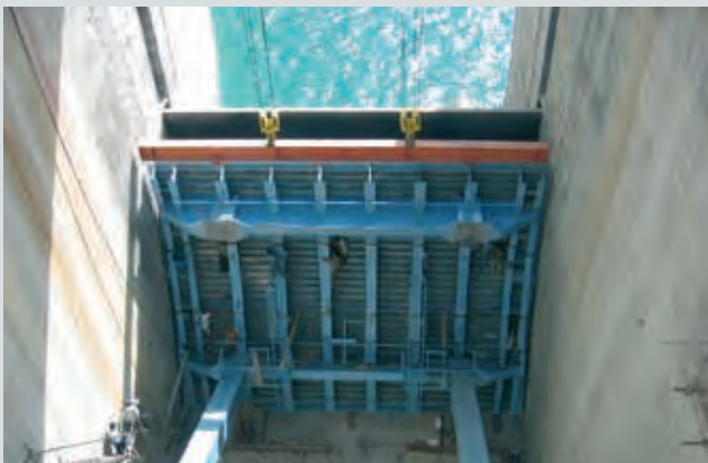
Segment geschlossen – Radial Gate closed
