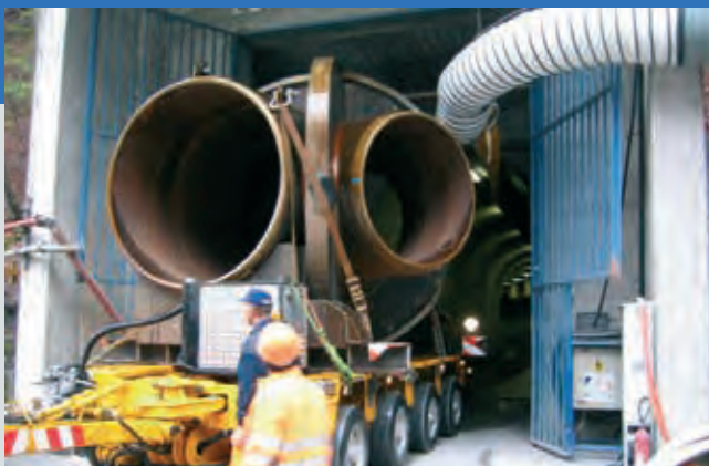
Transport des Hosenrohrs – Transport Bifurcator
