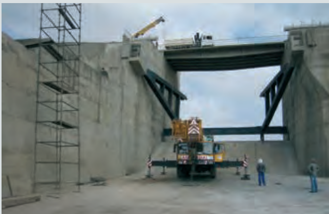
Montage Segmentschütz - Installation Radial Gates
