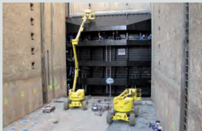
Hubtor - Vertical Lift Gate
