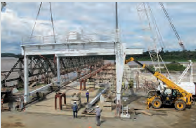
Kranmontage - Erection Gantry Crane
